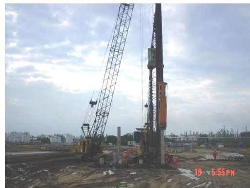
Fig 5. Pile driving
