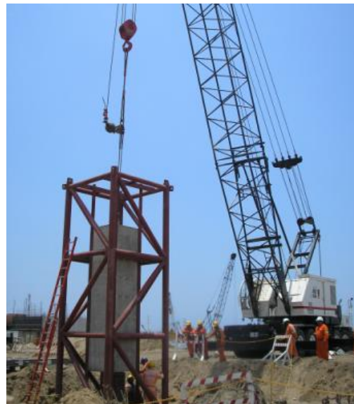
Fig 8. Dynamic tests for drilled shafts
