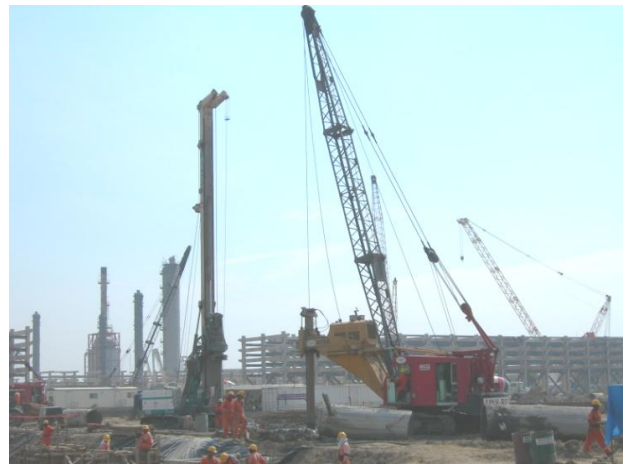
Fig 4. Drilled shaft construction
